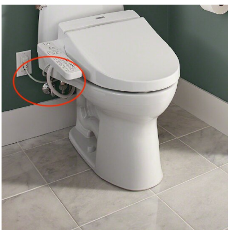
TOTO WASHLET – CORDS & HOSES ARE VISIBLE
